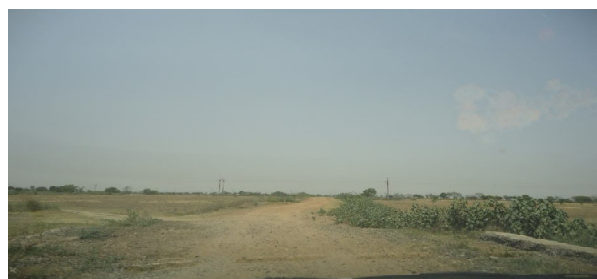
Road constructed Under MGNREGA, Damoh District, MP, May 2014
